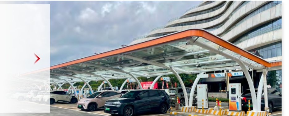
Petro China Guangxi V2G Charging Station
