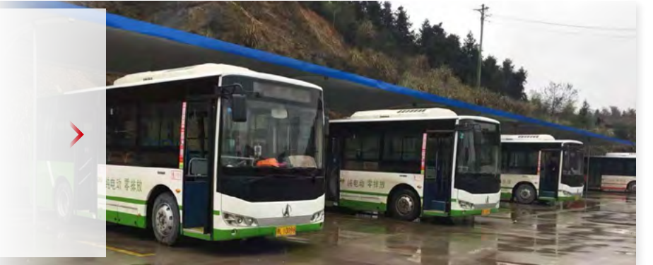
Hubei Bus Charging Station
